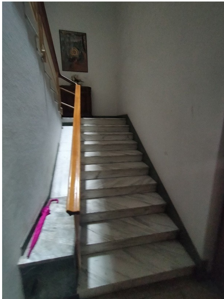
- RAMPE SCALE CONDOMINIALI -
